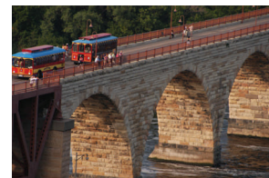
Stone Arch Bridge by MCC member Dave Lucas
